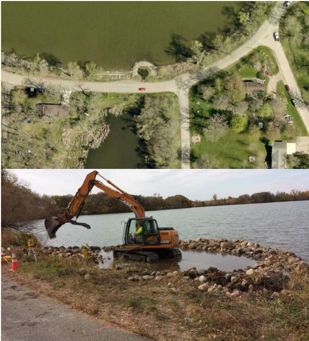
Figure 1. Example permeable rock berm fish barrier used in Iowa.
