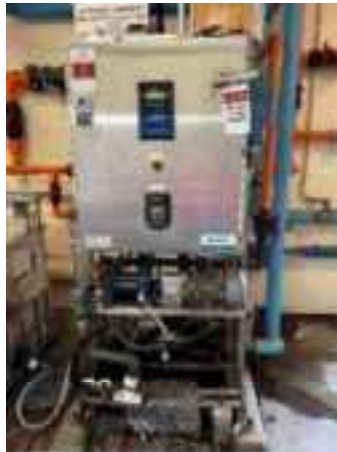
Figure 2-21: Polymer blending system
