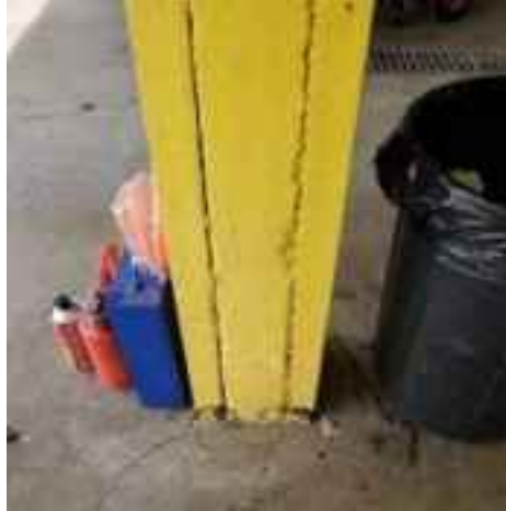
Figure 2-30: Loadout area column base
