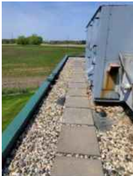
Figure 2-31: South roof edge by AHU
