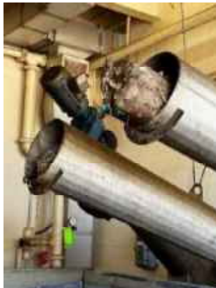
Figure 2-5: Screening compactor discharge
