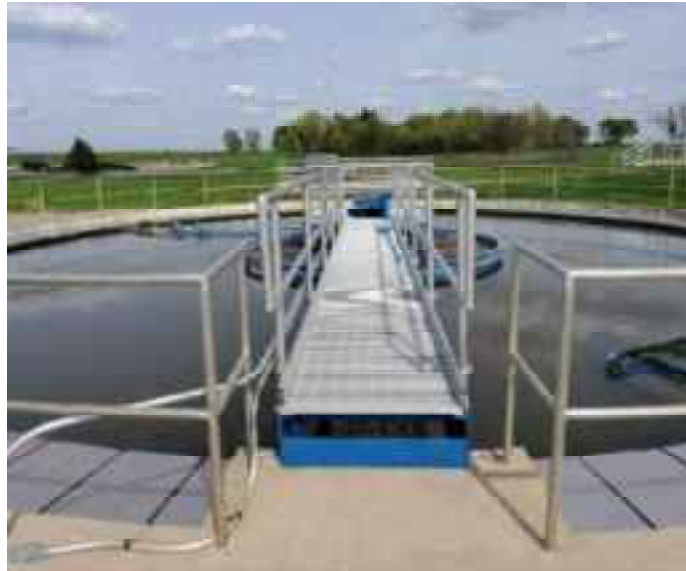
Figure 2-11: Secondary clarifier 2
