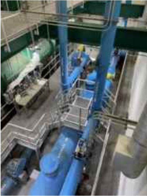
Blowers for Process and Membrane Air
