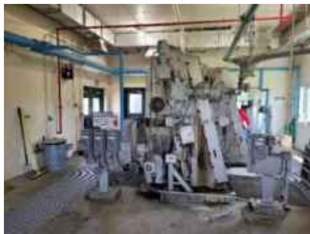
Figure 2-3: Perforated plate screen
