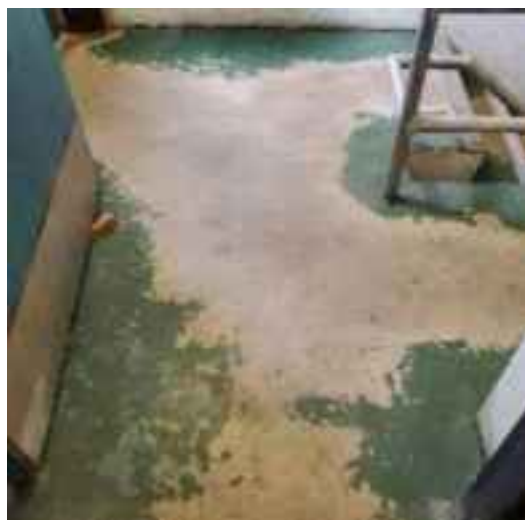
Figure 2-29: Painted floor near stairs in the loadout area
