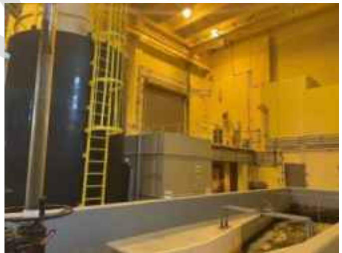
Odor control and UV channel
