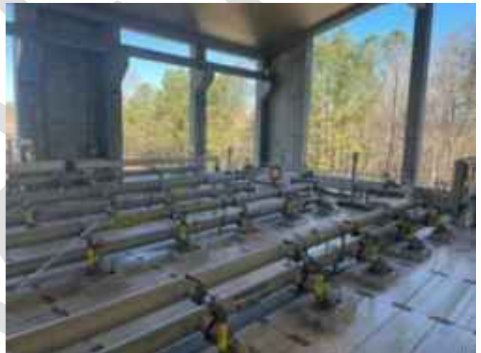
Membrane Tanks (Covered)
