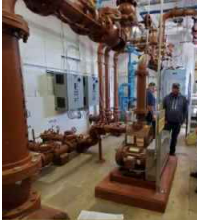
Figure 2-17: Recirculation pumps
