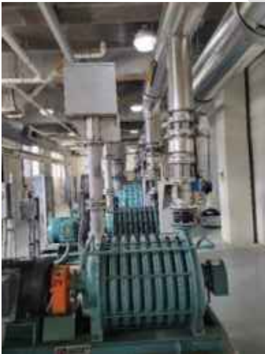
Blowers for Process and Membrane Air
