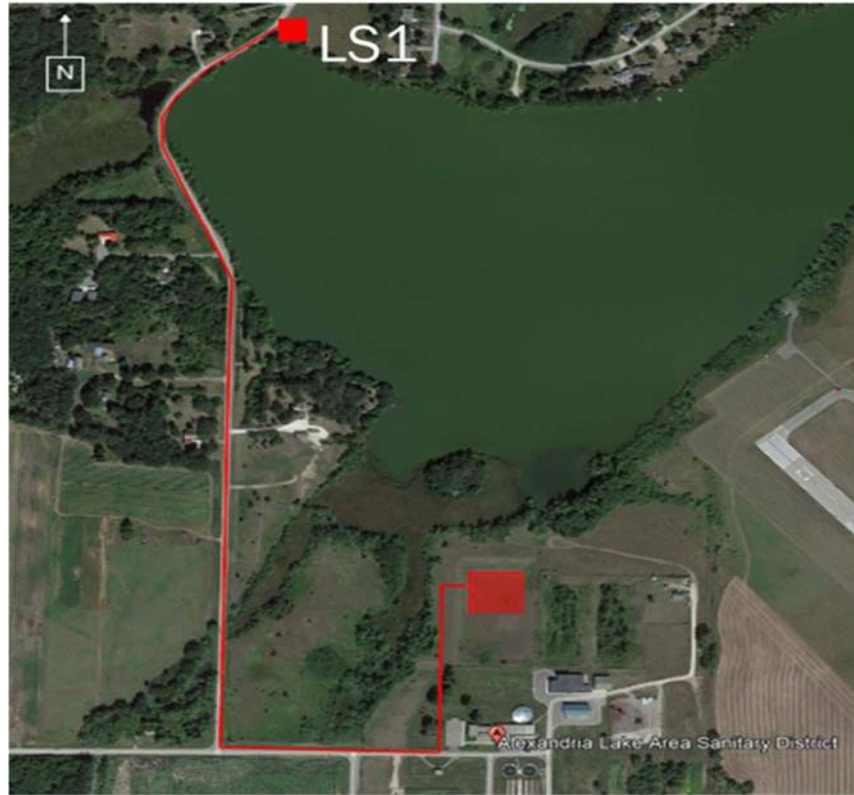
Figure 7-2. Proposed Forcemain from LS-1 to the WWTF EQ Basin for Peak Flows
